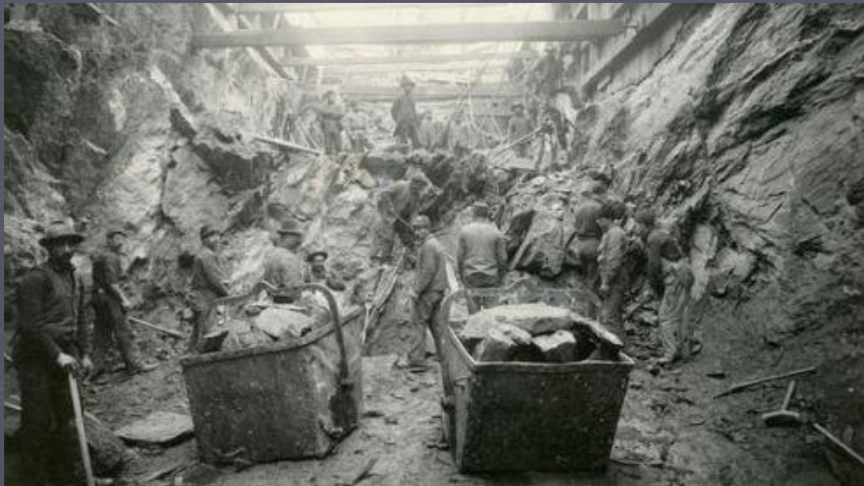
SUBWAY CONSTRUCTION (DECEMBER 1900)
